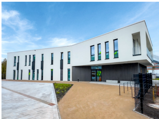
The exterior view of the new daycare centre at the TÜV NORD Campus in Essen.
